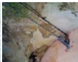
Shape Memory Alloy based device for the stabilization of the draught strength of vaulted masonry structures
