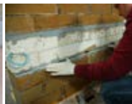
Strengthening and real time monitoring of a masonry structure with smart rebar
